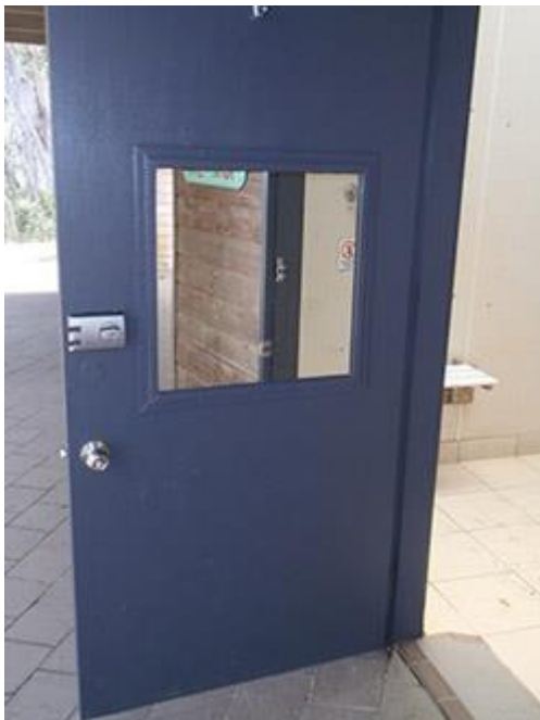
Entrance door to accessible toilet and shower
